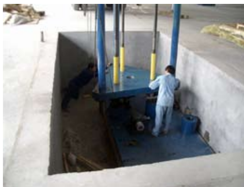
Mounting of the first press into its pit
