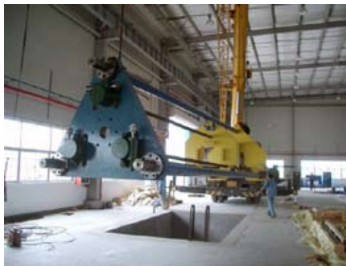
Overhead crane erects the press uprights
